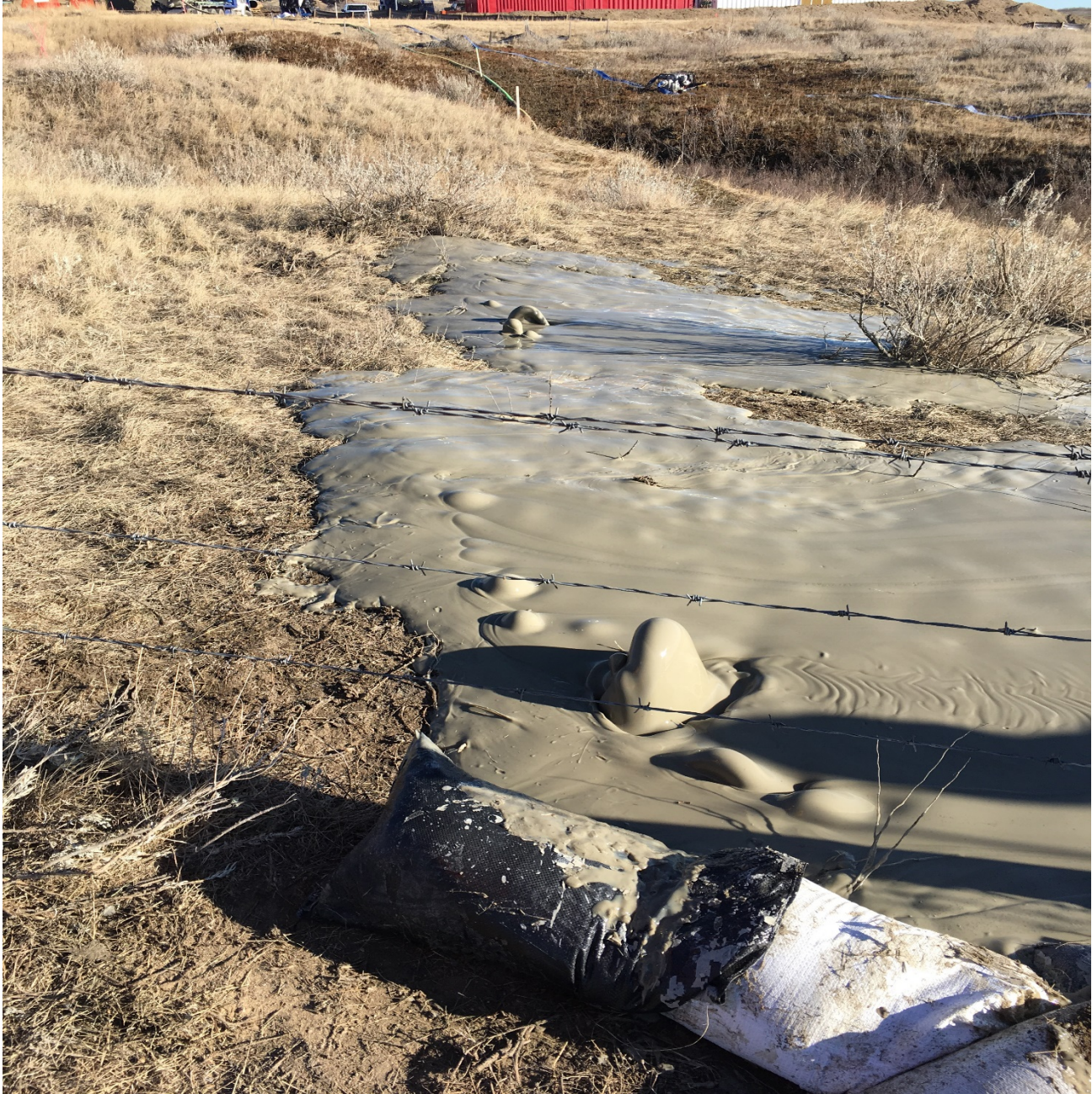
FRACK OCCURRING NEAR EXIT POINT.
