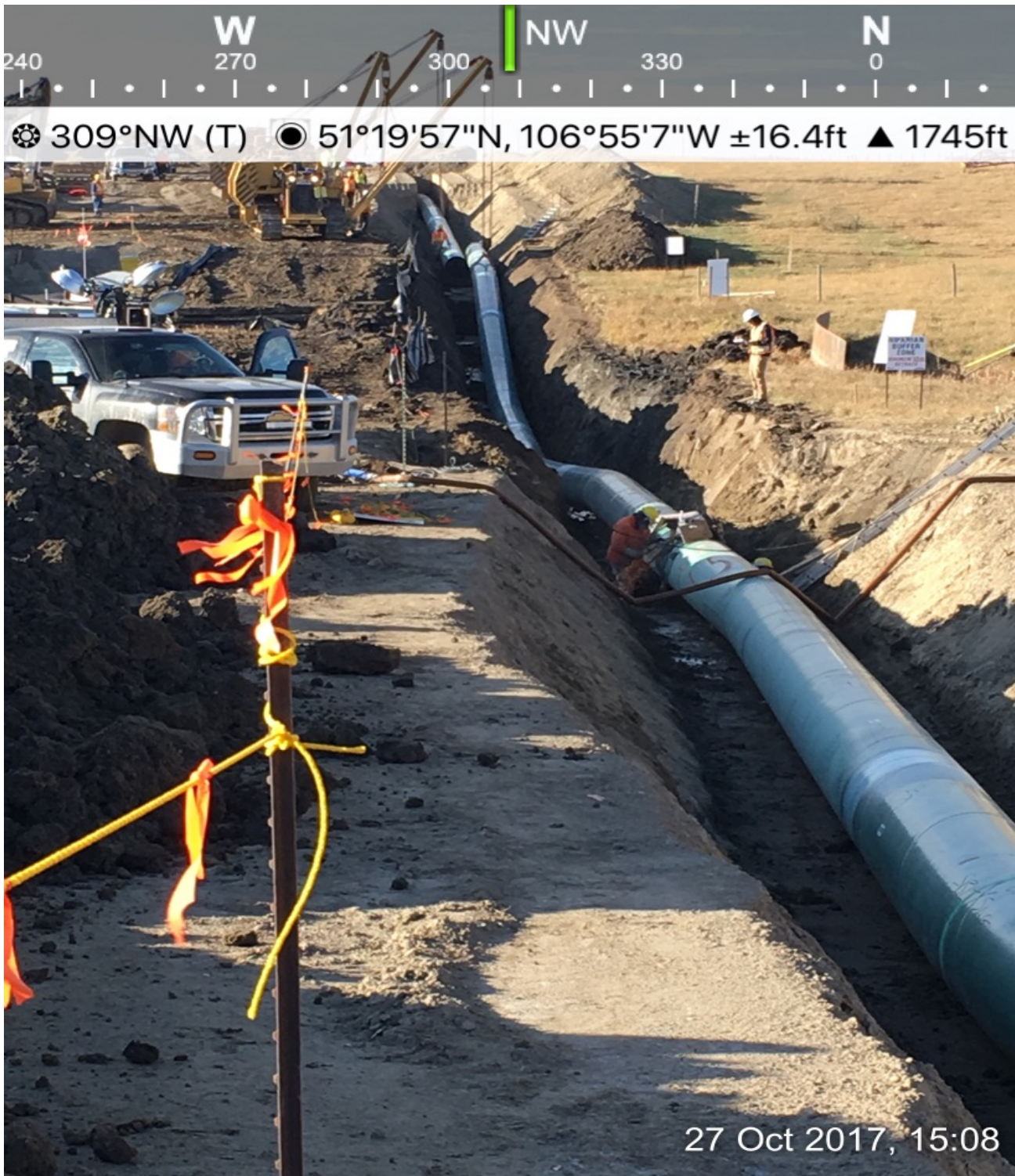
Welding up pipe at the creek crossing
