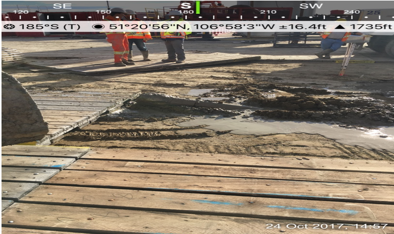
Pilot reamer of the horizontal drilling exit point at South Saskatchewan River
